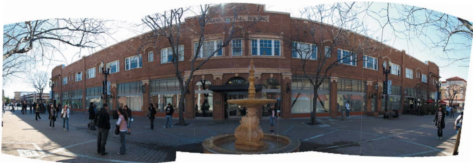
grand central building. directly across from proposed site.
